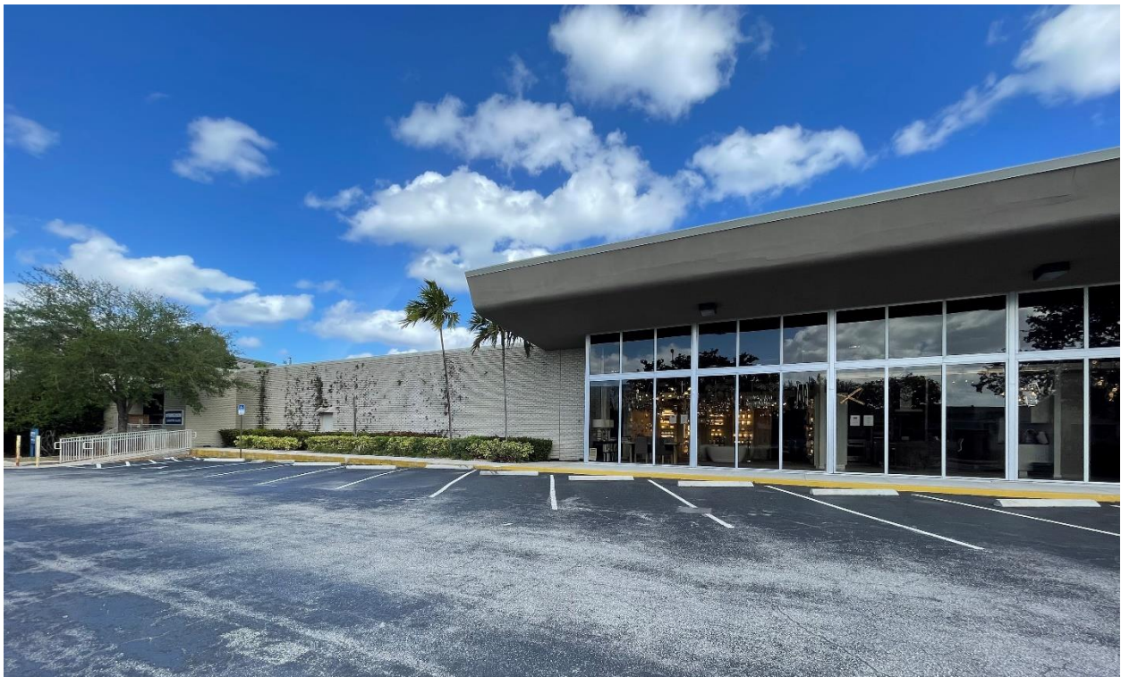
Front Elevation Looking Northeast
