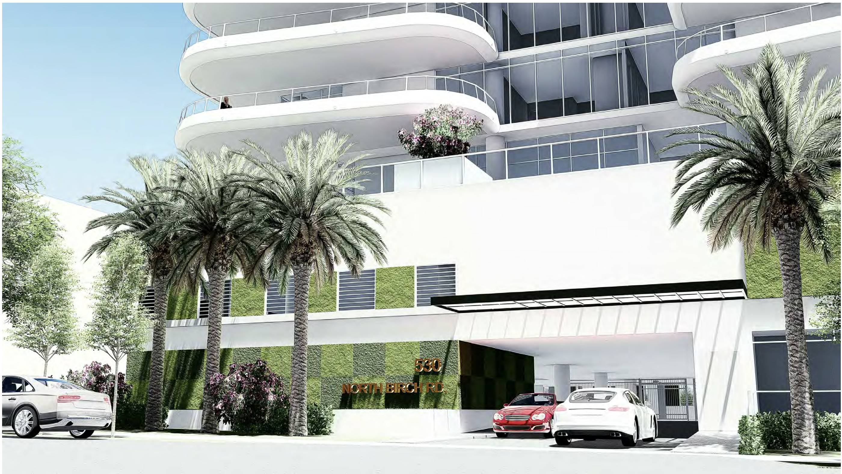
PARKING GARAGE ENTRANCE VIEW
