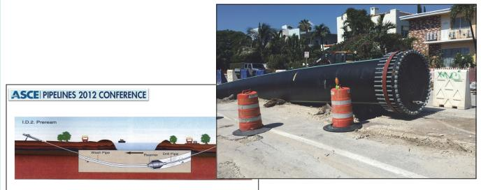
Emergency Relocation of 20-Inch Sewer Force Main (HDD)
