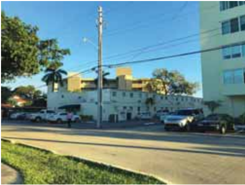
NORTH WEST CORNER VIEW
