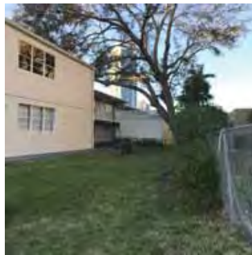
EAST BACK VIEW
