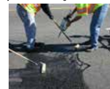
Fig. 5 Squeeze out sealer and spread with roller.
