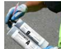
Fig. 4 Prepare sealer cartridges for use in sealer gun.
