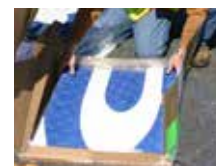
Fig. 1 Handle sheets with plastic
