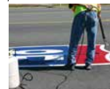
Fig. 7 Heat PreMark material
