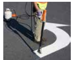
Fig. 3 Heat PreMark® material according to instructions.
