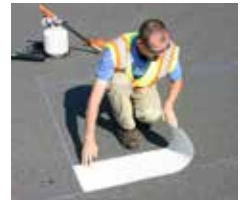
Fig. 2 Position PreMark® material according to diagram provided
