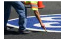
Fig. 2 Position marking to draw outline of application area
