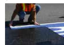
Fig. 6 Position PreMark® material according to diagram provided.
