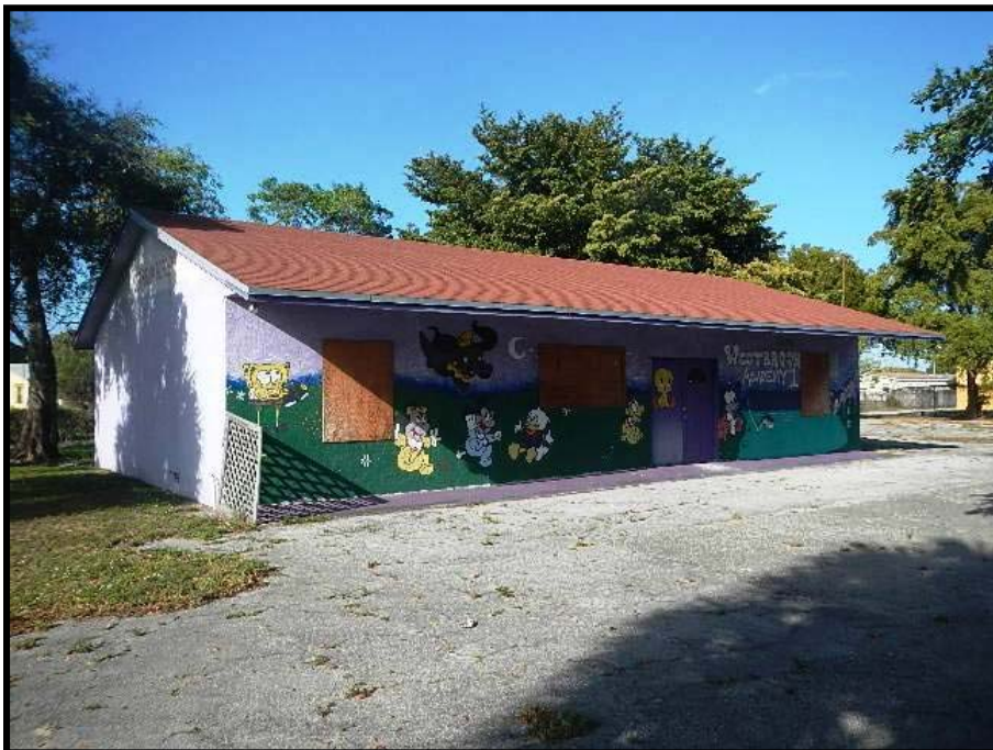
Below: 2. Front View of Subject
