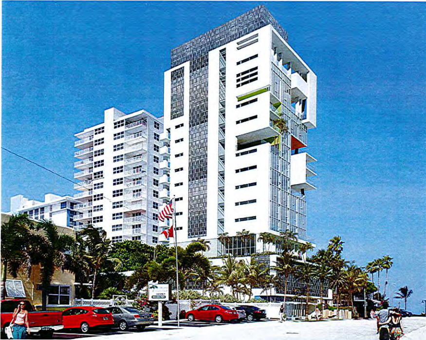
C1 VIEW FROM ALHAMBRA STREET LOOKING NORTHEAST
