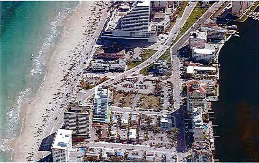
A1 AERIAL VIEW LOOKING SOUTH
