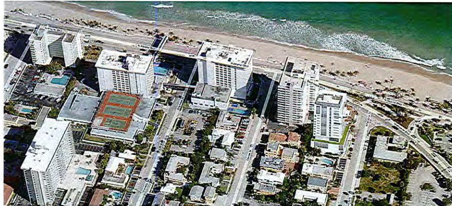
A4 AERIAL VIEW LOOKING EAST
