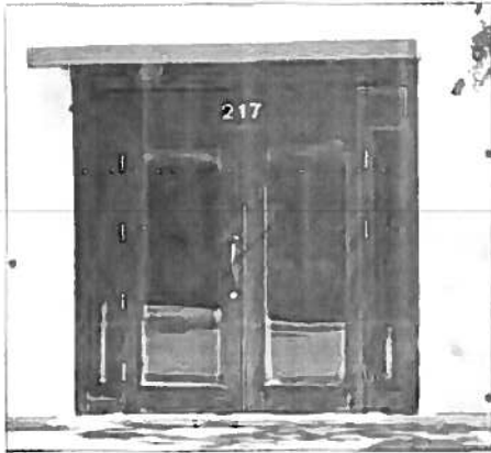
Entrance doors typically include glass and were often paired historically.
