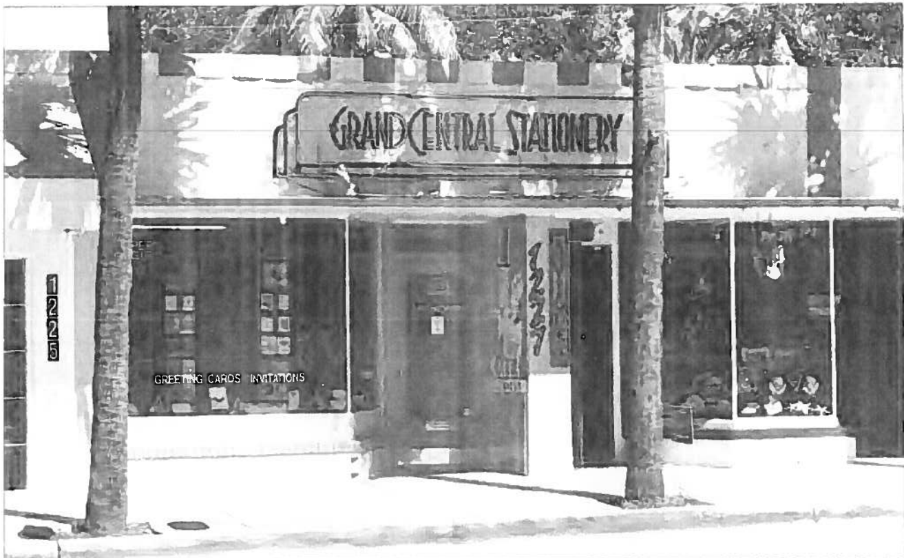
This storefront includes large display windows, a entrance alcove with a wood, single-light door topped by a transom window, a customized neon sign and a unique paint scheme that complements its architectural style.
