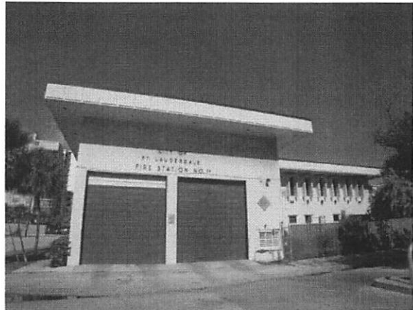
Looking Northeast at Building Rear
