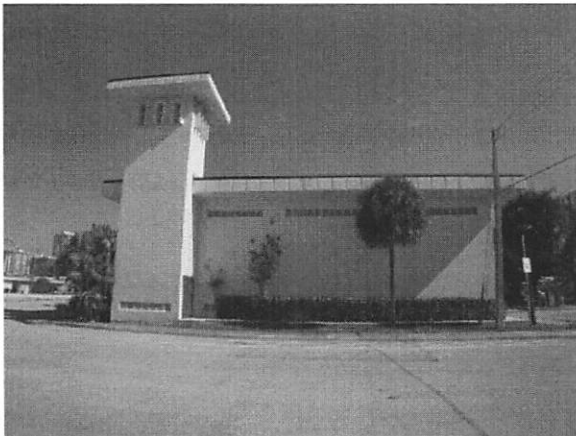
Looking East at West Elevation
