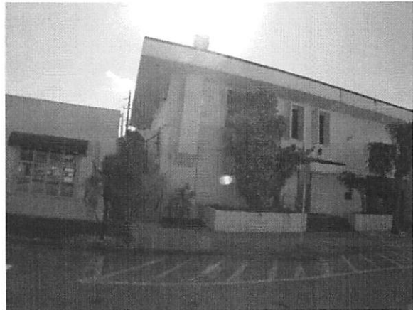
Looking Southwest at East Elevation
