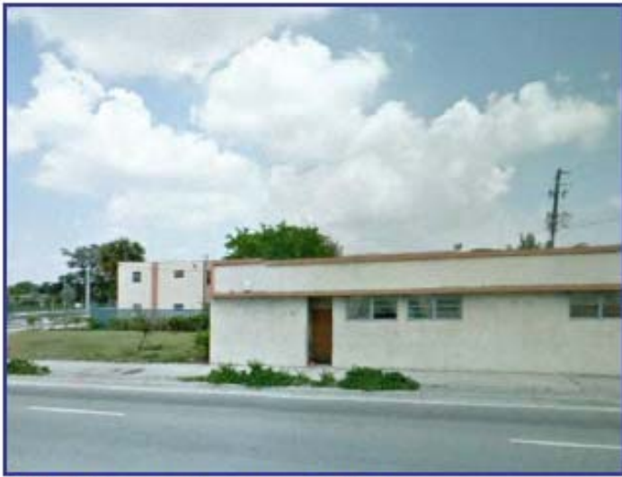
915 Sistrunk Boulevard, Before
