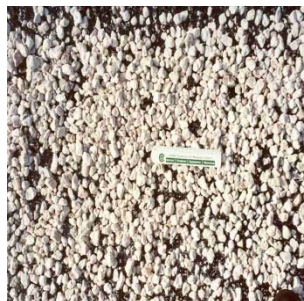
Figure 6 - Completed ARMI/Rubber Modified
