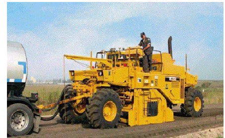
Figure 4 - Full Depth Reclamation (FDR) Base
