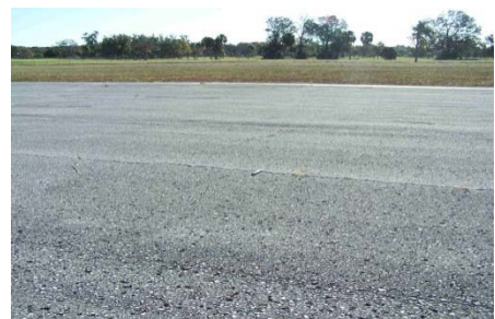
Figure 2 - Corrugation (Ripple) Distress
