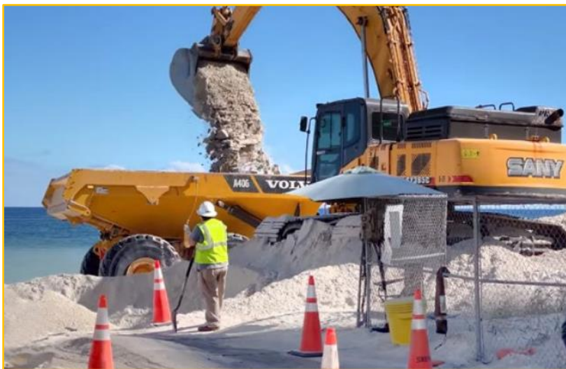
Beach renourishment on Fort Lauderdale Beach
