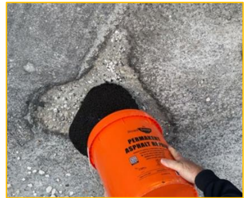
Application of Road Soup's asphalt repair product
