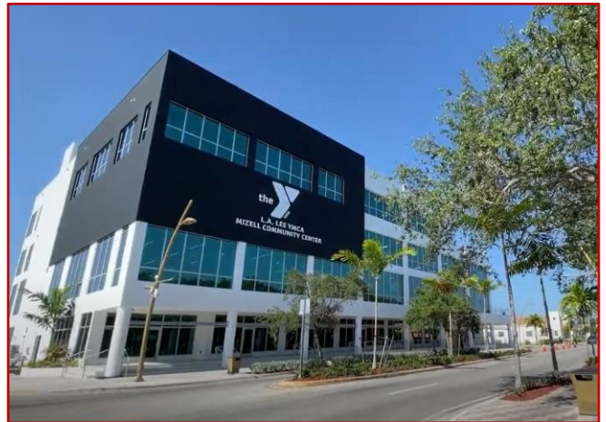
Recently completed LA Lee YMCA/Mizell Community Center
