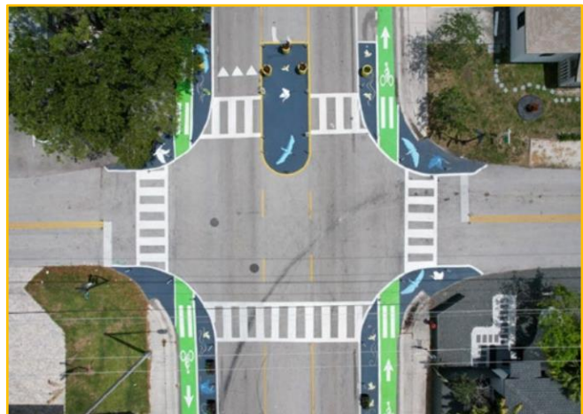
NE 15th Avenue after improvements
