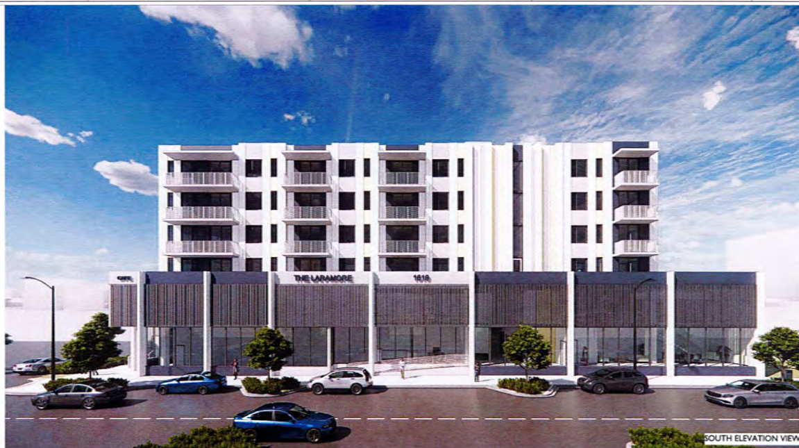
SOUTH ELEVATION VIEW
