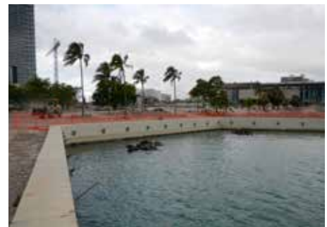
Bicentennial Park seawall
