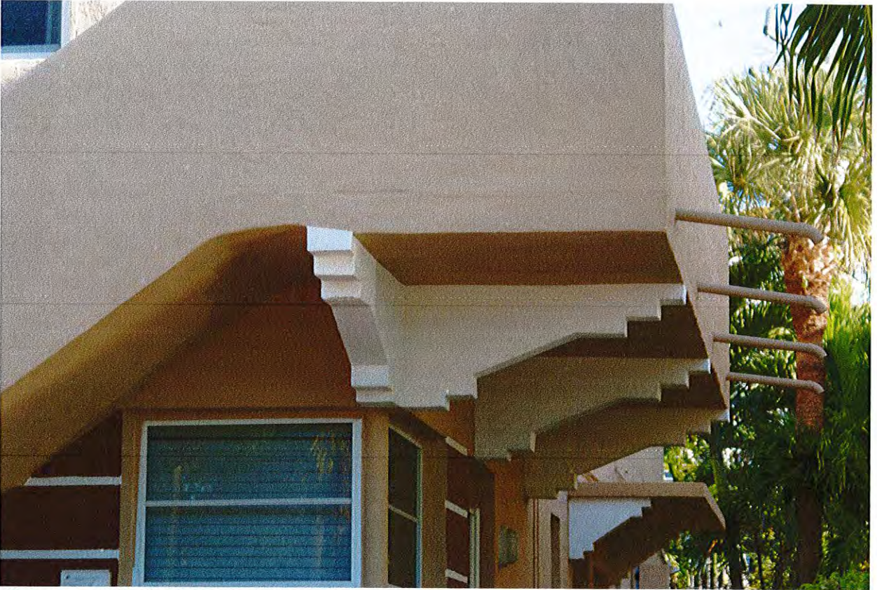
Close-up of Stylized Brackets Supporting Staircase
