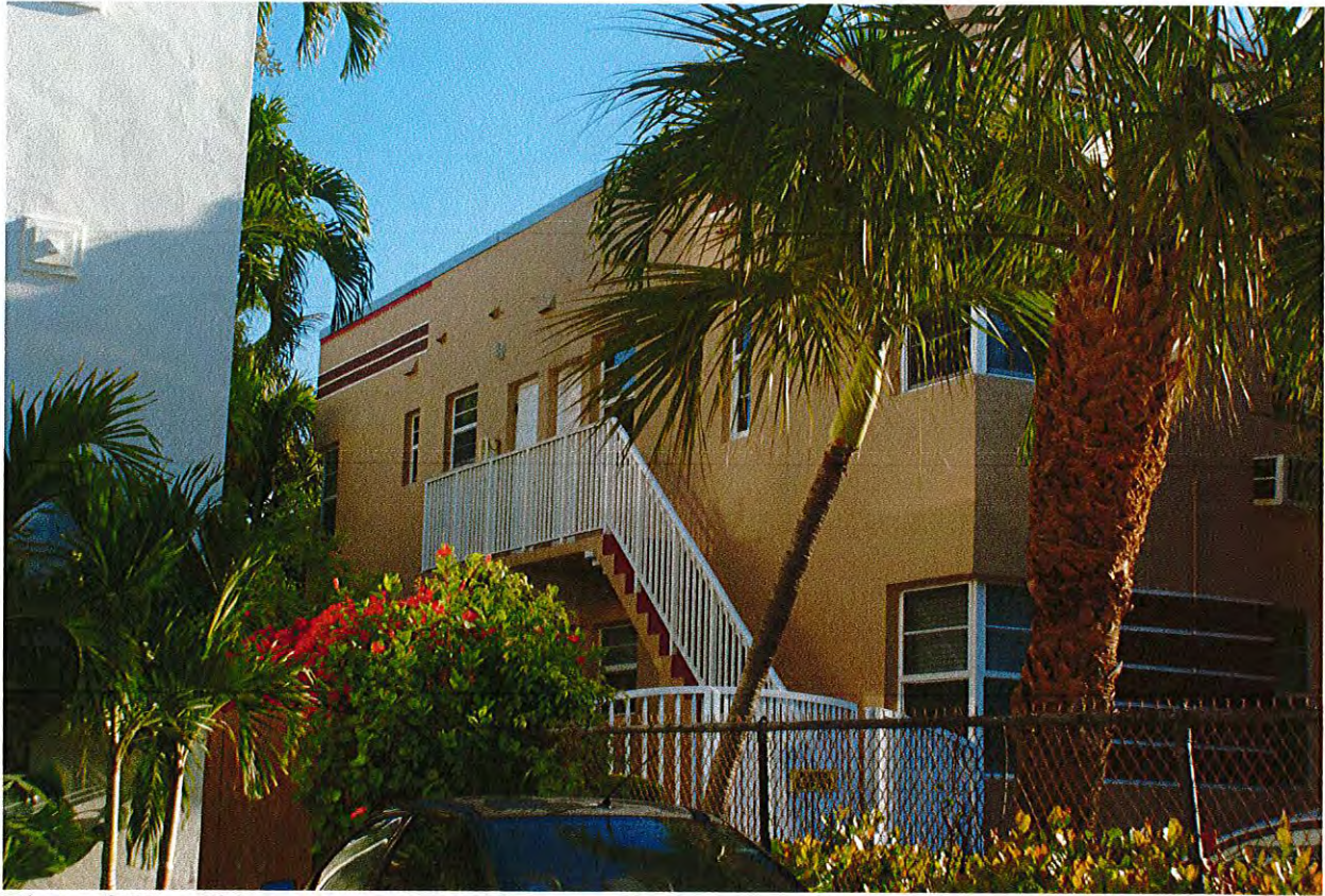
View of West Side
