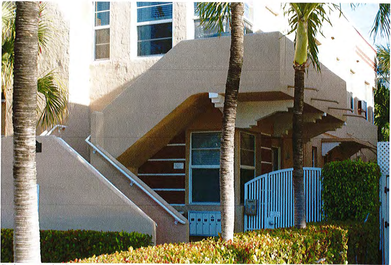
Staircase to the Second Floor at the Southwest Corner
