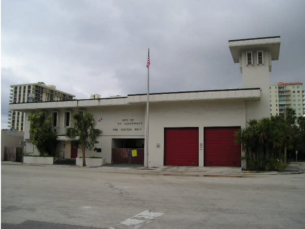
VIEW SOUTHERLY FROM ACROSS NE 32 ST.
