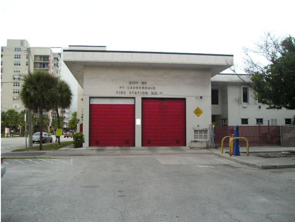
VIEW NORTHERLY OF SUBJECT PROPERTY FROM ACCESS ROAD ENTRANCE
