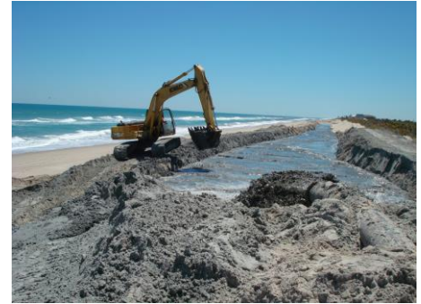
Beach placement of inlet trap sand
