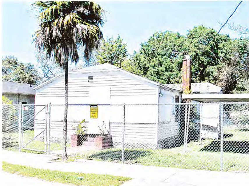
521 NW 13 AVENUE LOOKING SW FORT LAUDERDALE, FLORIDA
