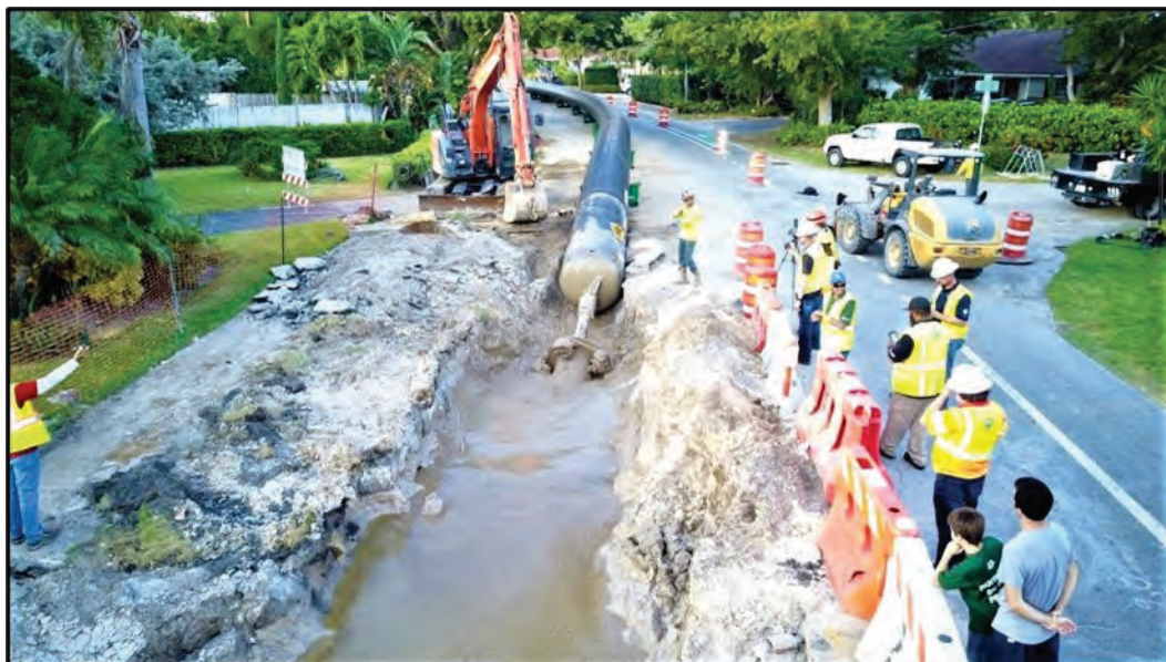
48" HDD in Fort Lauderdale
