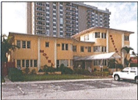
Fort Lauderdale's hotels and motels were constructed in a variety of styles including this Art Moderne example. Note the projecting roofline and wrapping corner windows.
