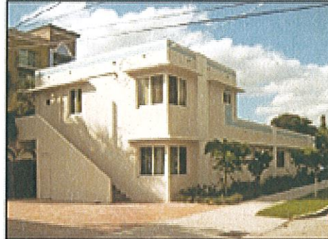
This Art Moderne building has a 2-story main block with a 1-story wing visually joined by with a decorative band. Windows wrap around corners and are covered by cantilevered sun screens.
