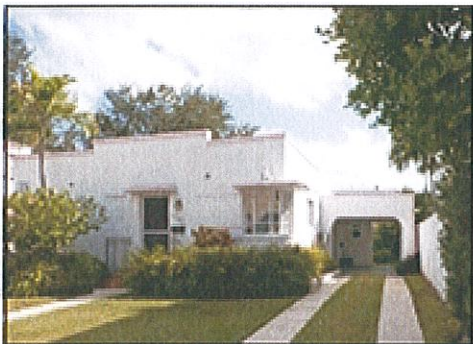
This Art Moderne residence has a central projecting parapet topped by a coping, corner wrapping windows with cantilevered sun screens, and a smooth stucco surface with horizontal grooves.
