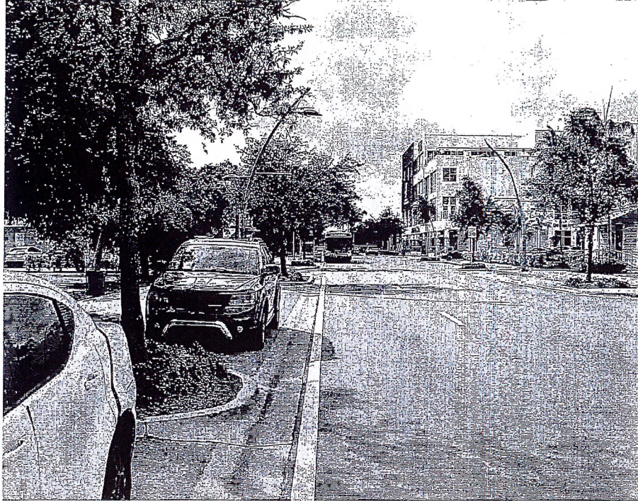
NW 6 STREET, LOOKING WEST
