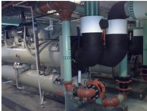
(2) Newer 150ton High Efficiency
