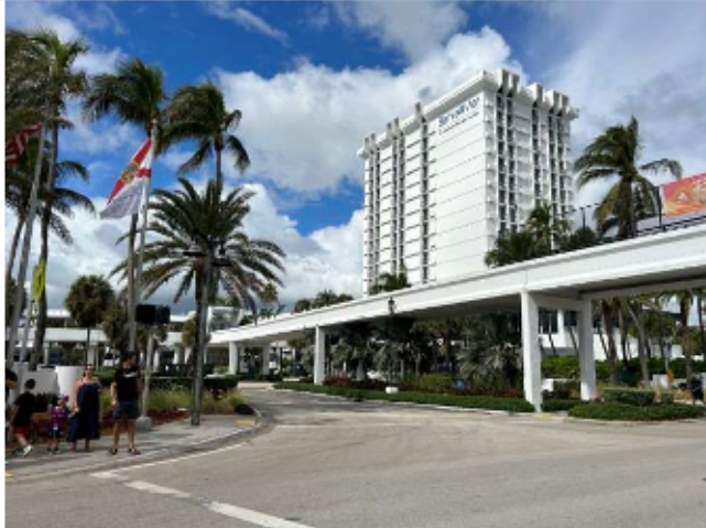
Current Improvements on Site Looking West
