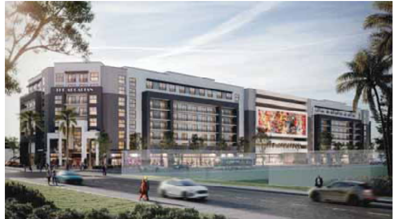
02 - CONTEXT VIEW FROM NORTH WEST
