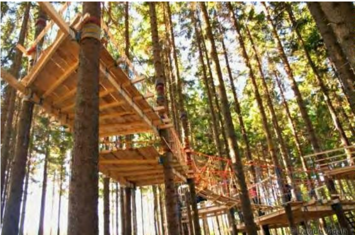
Lashed wood tree-walk platforms
