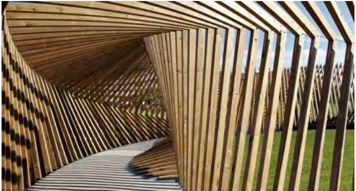
Natural volumes formed using stock wood planks
