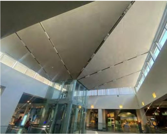
View of atrium ceiling
