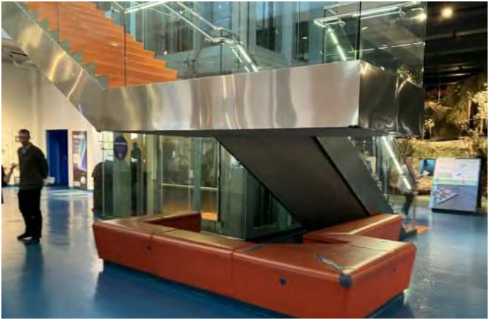
Lower stair landing
