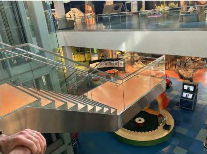
2nd floor to upper stair landing
