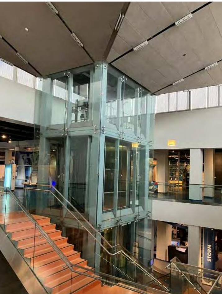
Elevator shaft from 2nd floor
