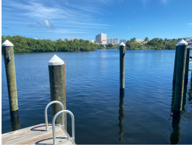
1. Subject site, showing the existing mooring pilings.
