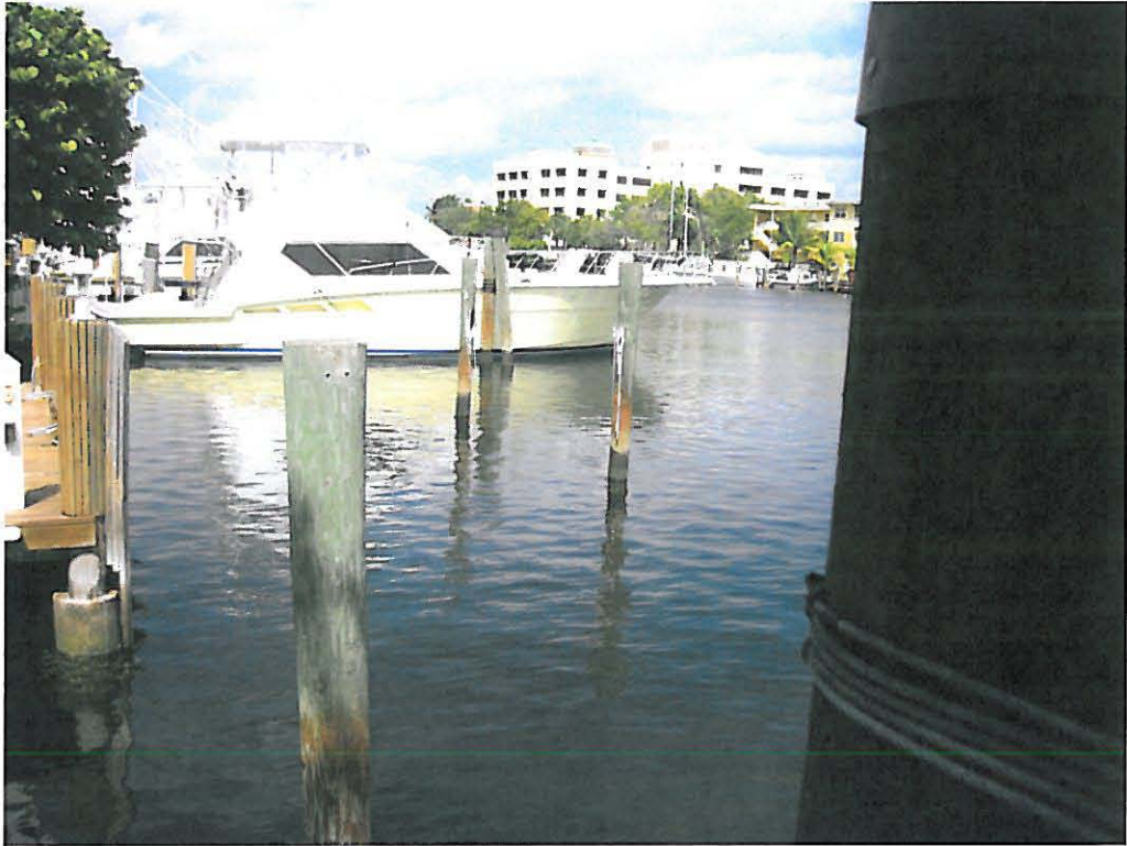
1. Northern property boundary, facing north.
