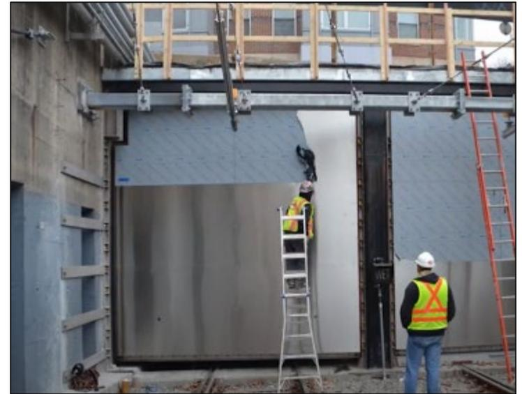
Figure 35: Floodgates Installation
