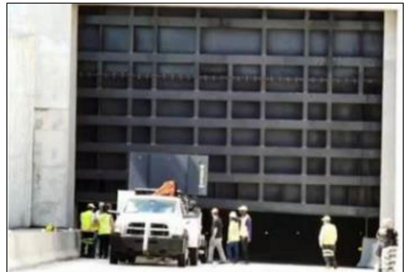
Figure 34: Flood Gates Mid-Closing at Port of Miami Tunnel
