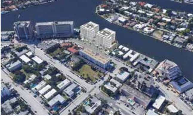
OBLIQUE VIEW - FROM THE NE
