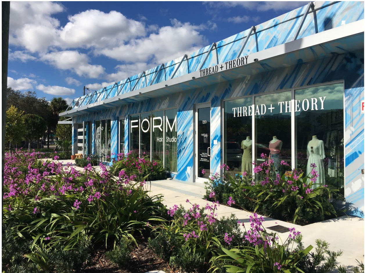
Completion of the Fabrik Project at 801, 80, 815 and 819 NW 2 Avenue in Progresso Village.
