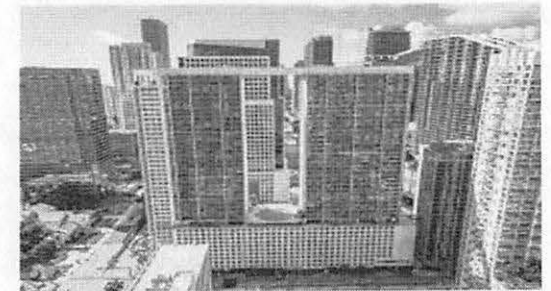
Repairs and Retrofits Brickell 500
