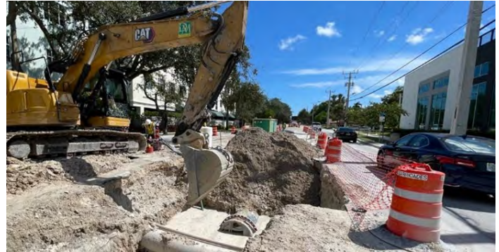
Arcadis CEI Project - Preparation work for utility crossing under stormwater pipe
