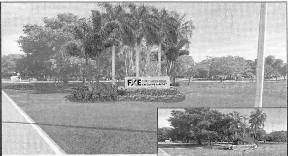
New Monument Signage and Landscaping at Main Entrances, like NW 21st Avenue, Elevates FXE's Brand in the Community
