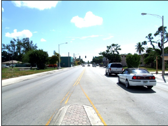
Figure 3.3, Sistrunk Boulevard/NW 6th Street Prior to Corridor Improvements
