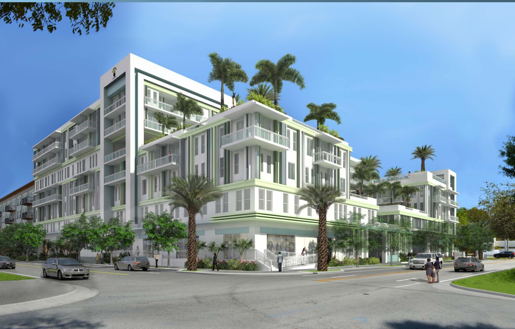
South Western Facade
