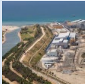
Hadera Membrane Plant IDE Technologies Hadera, Israel
