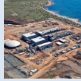
CITIC Cape Preston Plant IDE Technologies Cape Preston, Australia
