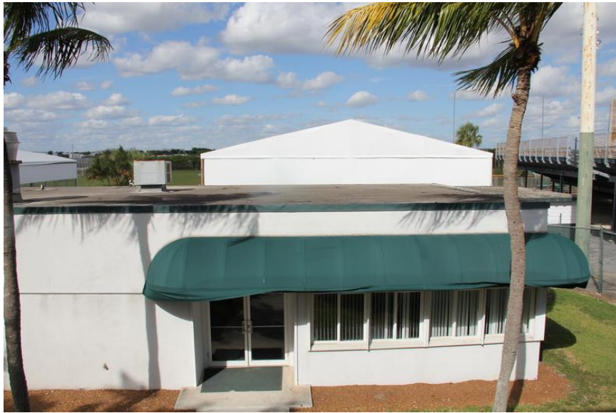
Overall view of Hospitality Building.
