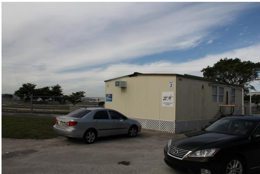
Overall view of Hut #2.
