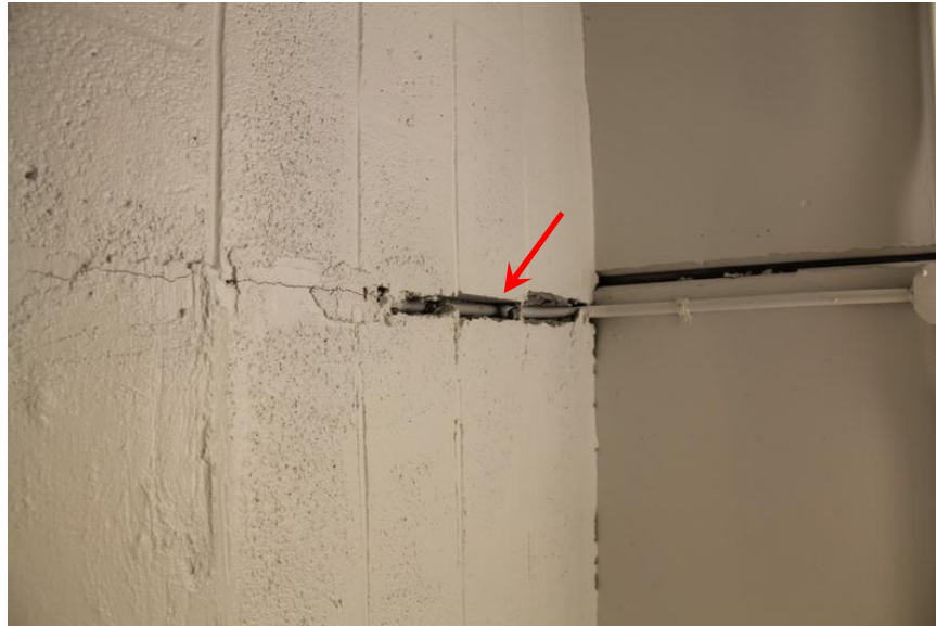
View of wall opening at the inset electrical conduit location.
