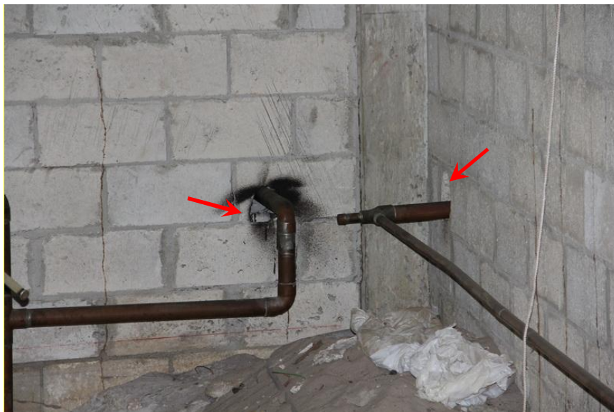
Typical view of pipe penetrations.
