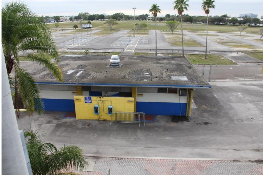
View of building roof.
