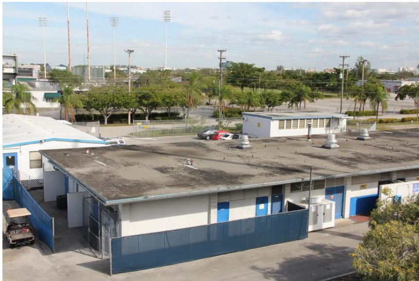
Overall view of the locker room building.
