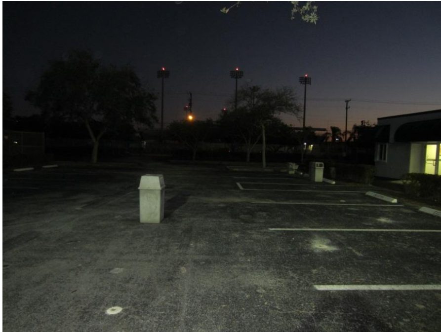
View of administration building parking lot; lighting level does not cover entire parking area.
