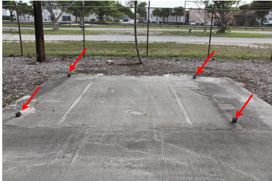
View of typical anchored metal brackets in the concrete slab.
