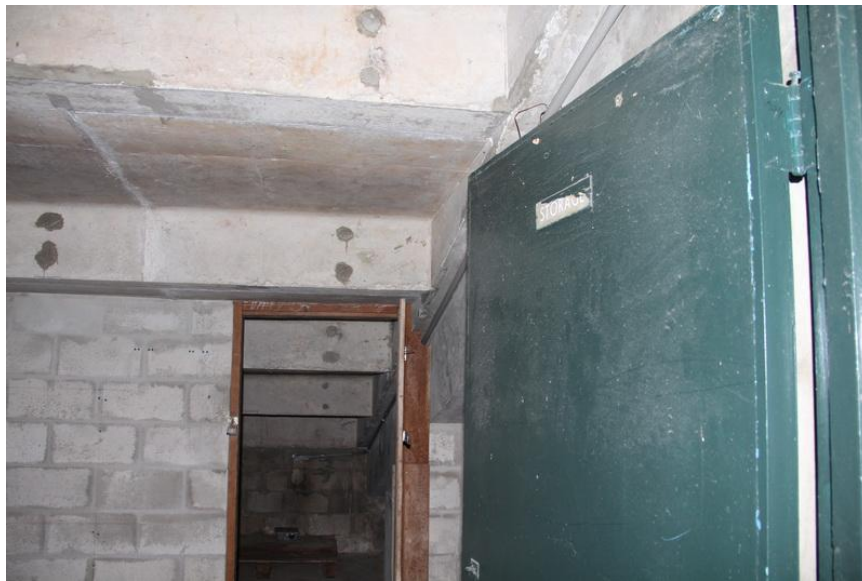
Overall view of Storage Room
