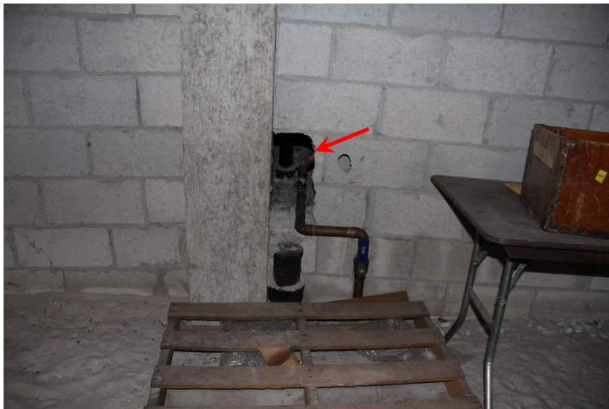
View of open wall penetration.
