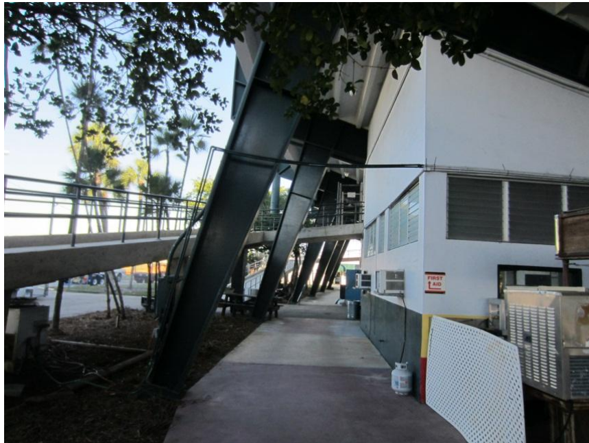
View of conduit not properly supported as required, conduit is sagging. This is located underneath the main stadium seating to the left of the main concession stand.
