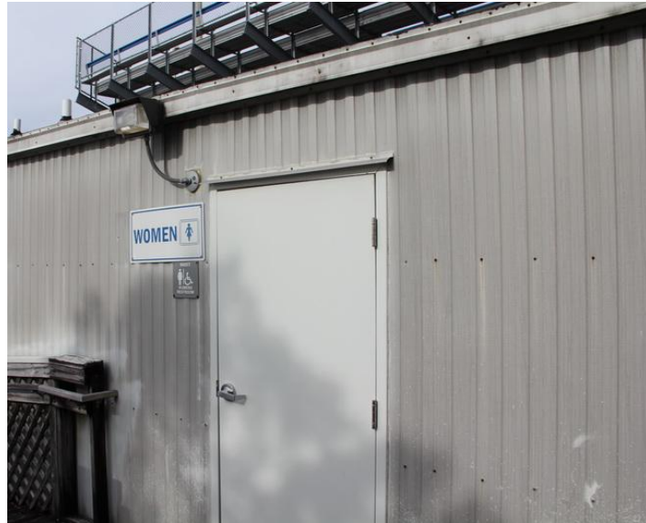
View of Building 1406T.
