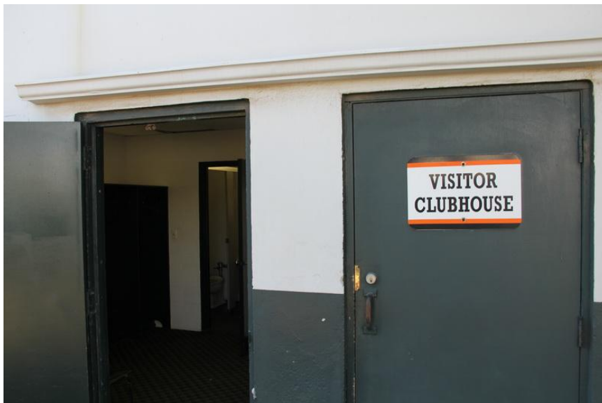
View of Visitor Clubhouse Entrance.
