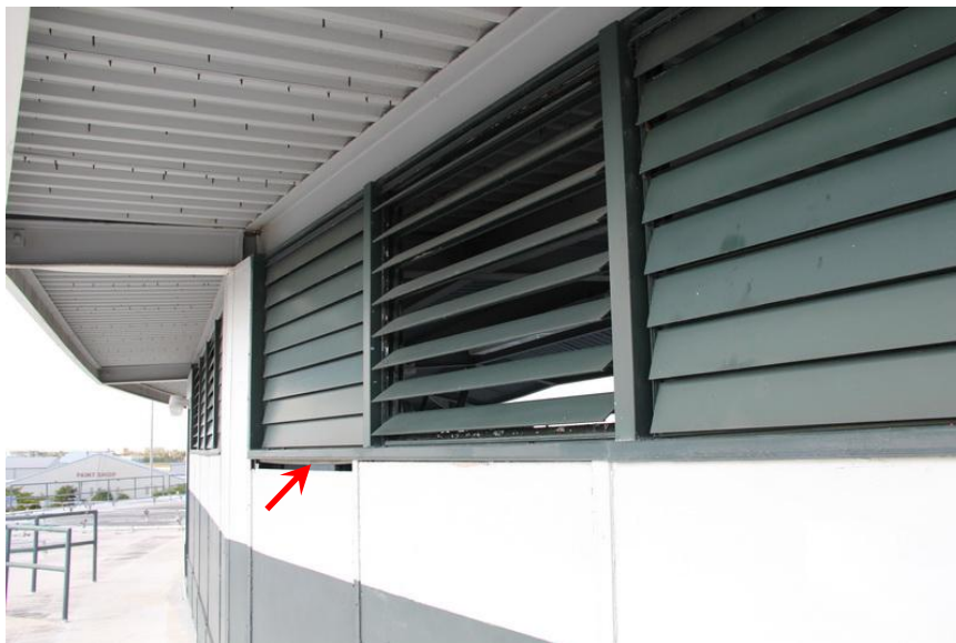
View of incomplete wall.
