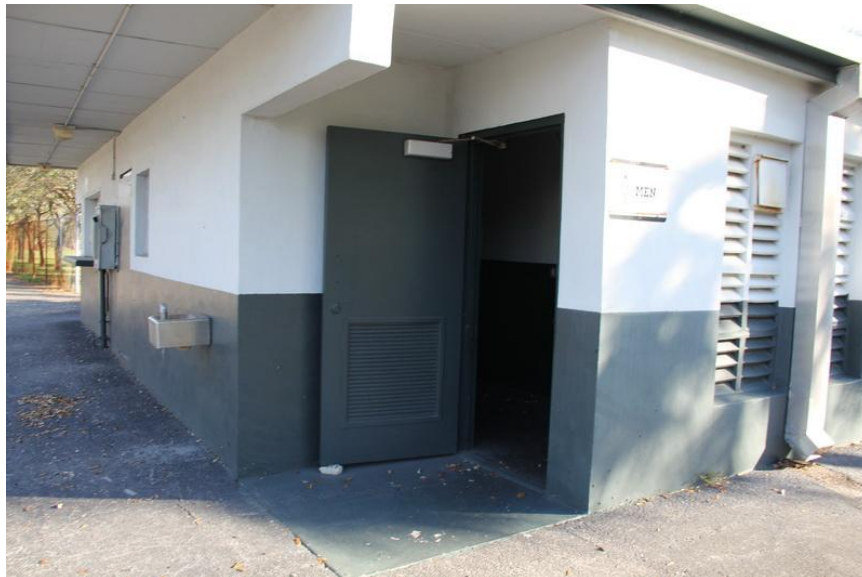
View of Right Field Concessions Building.
