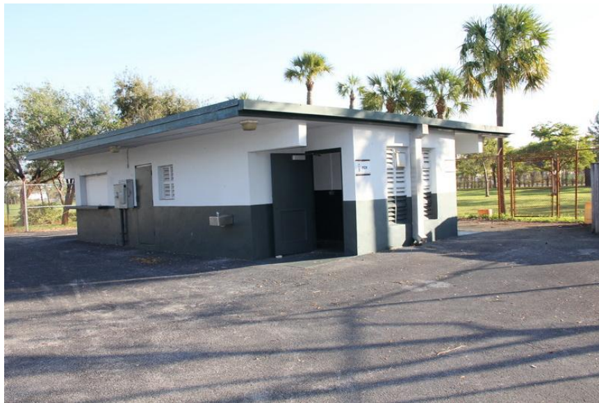
Overall view of Outfield Concessions Building.
