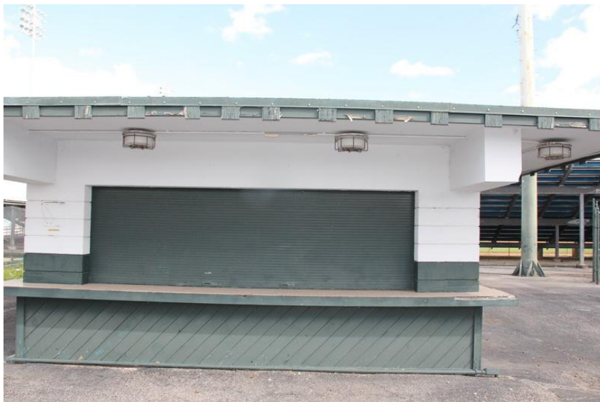
Overall view of Left Field Concessions Building.
