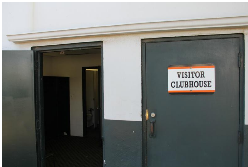
View of Umpire Room Entrance
