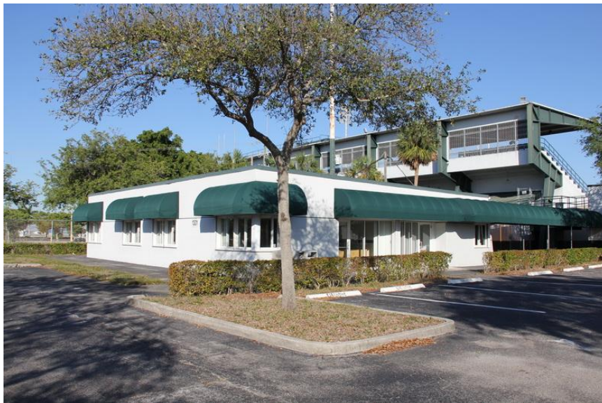
Overall view of the Administration Building.
