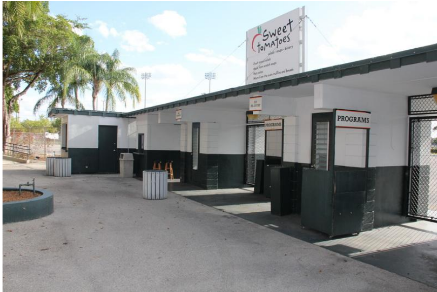
Overall view of Left Field General Admission Building.
