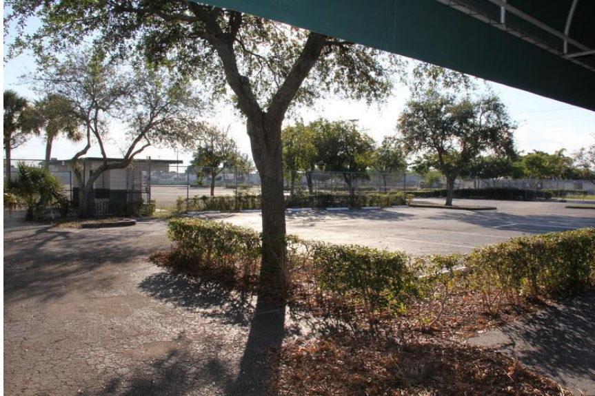
Overall view of Right Field General Admission Building.
