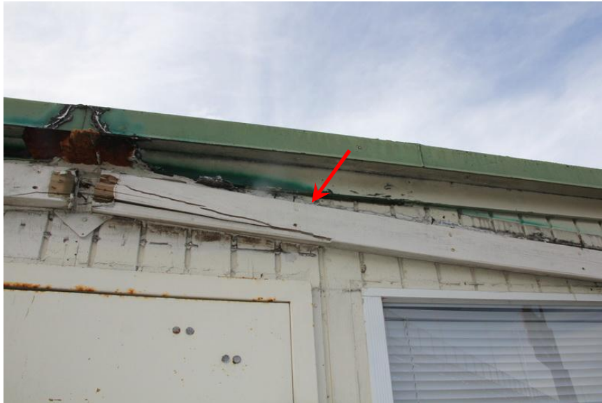
View of door overhang.
