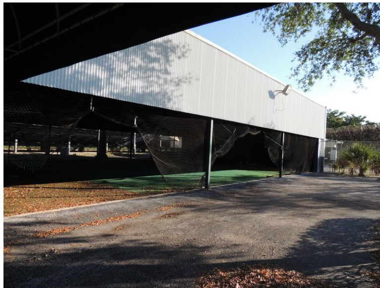
View of the Right Field Bullpen Building.
