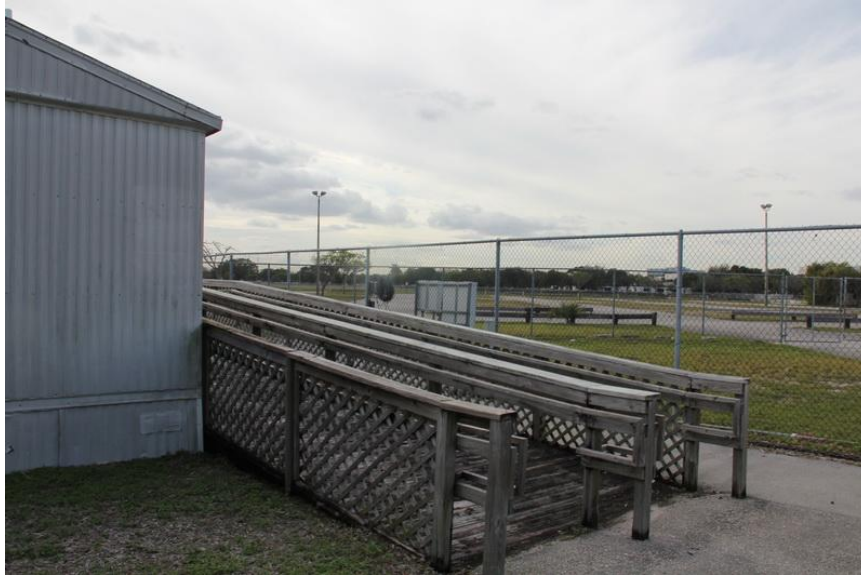
View of overall Building 1405T and Ramp.
