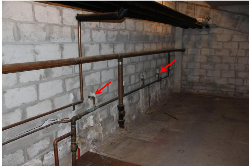
Typical view of pipe penetrations
