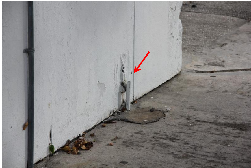
View of pipe penetration.
