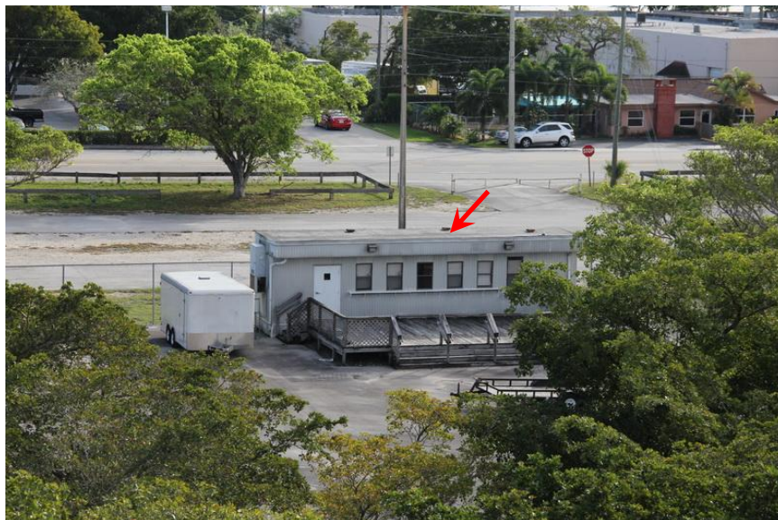
Overall view of Southeast (SE) Office.
