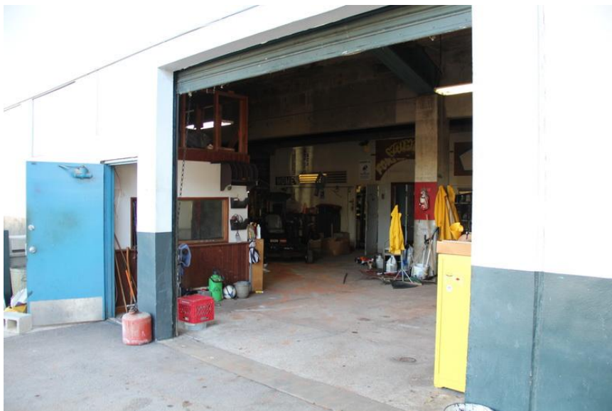
Overall view of Maintenance Facility.
