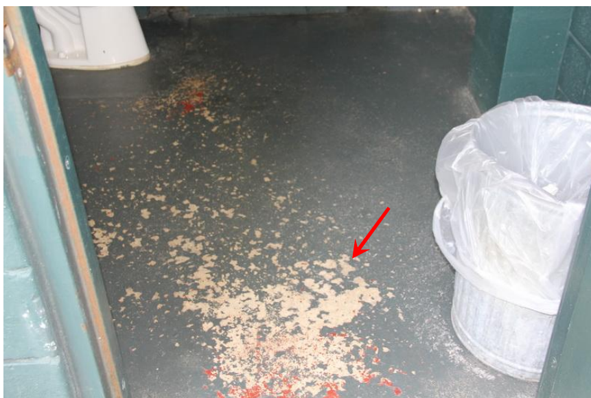
View of restroom floor.
