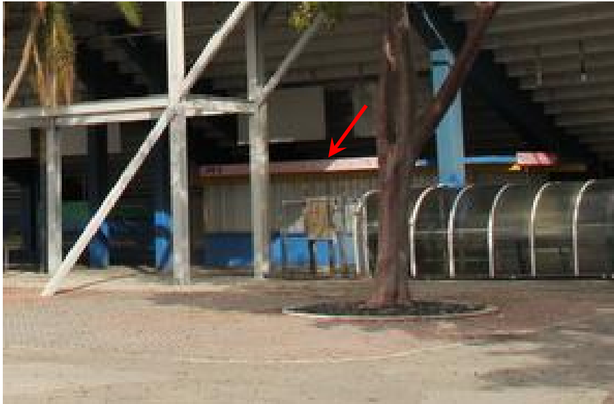
Overall view of South Concessions.
