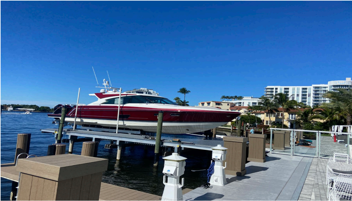
3. Southern portion of the subject site, facing northwest.
