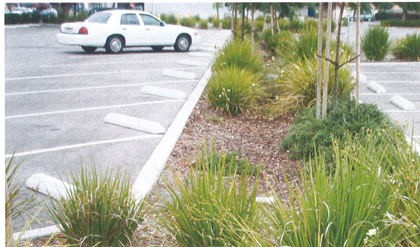
Flush Curb to Allow for Maximum Sheet Flow
