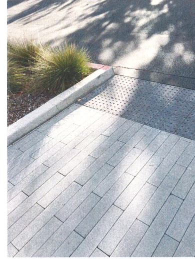
Detection Warning Pavers
