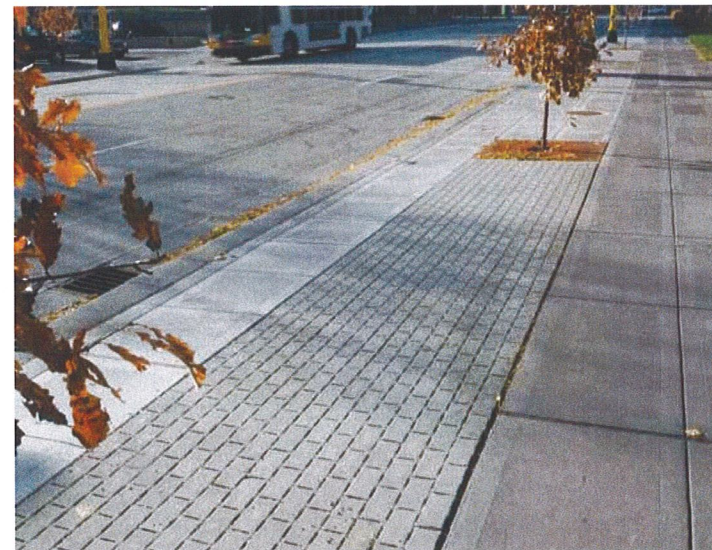
Pervious Paver Parking
