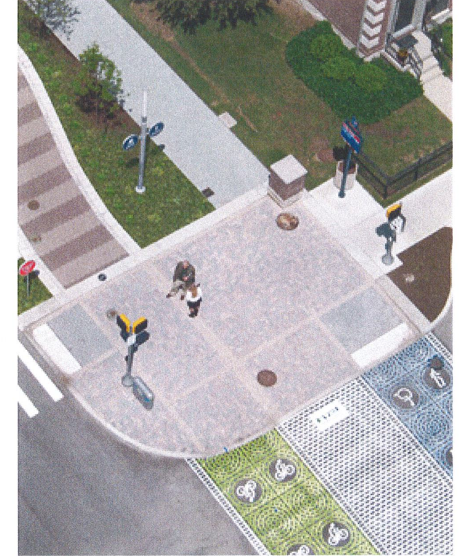
Crosswalk with Bike & Pedestrian Delineation
