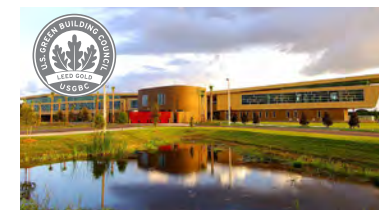
Hillsborough Community College Multipurpose SouthShore
