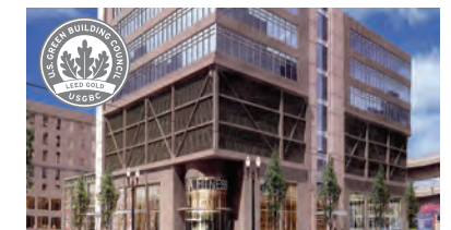
Machine Works LLC Machine Works Building
