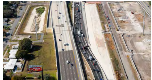
I-275 Reconstruction Tampa, Florida
