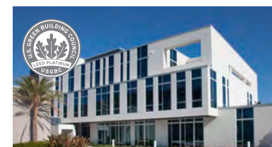
City of Miami Gardens - seeking LEED® Platinum Certification
