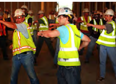
Skanska requires Stretch and Flex on our jobsites every morning
