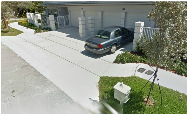
A mistake in the design and permitting process led to an offset sidewalk to route pedestrians around vehicles in a too-short driveway 1700 block of 5th Pl
