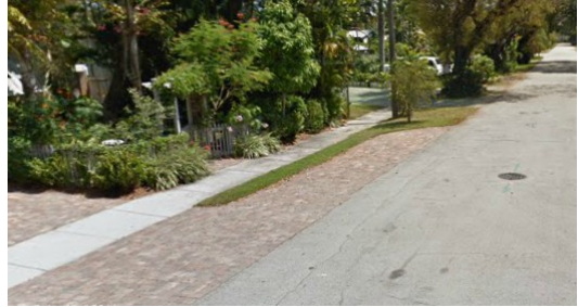
Pavers — Driveway Apron and Swale 700 block NE 18th Avenue
