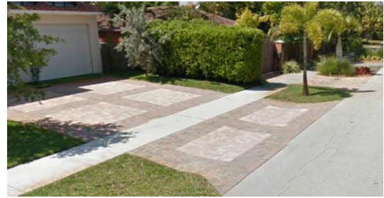
Pavers — Driveway Apron 500 block NE 13th Avenue
