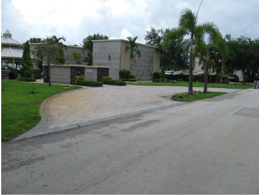
Existing Mausoleum Buildings – looking northwest towards existing circular drive.
