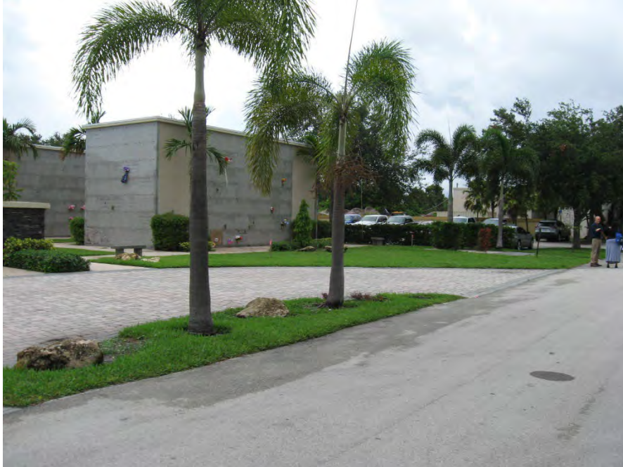
Existing Mausoleum Buildings – looking northwest towards NE existing building.
