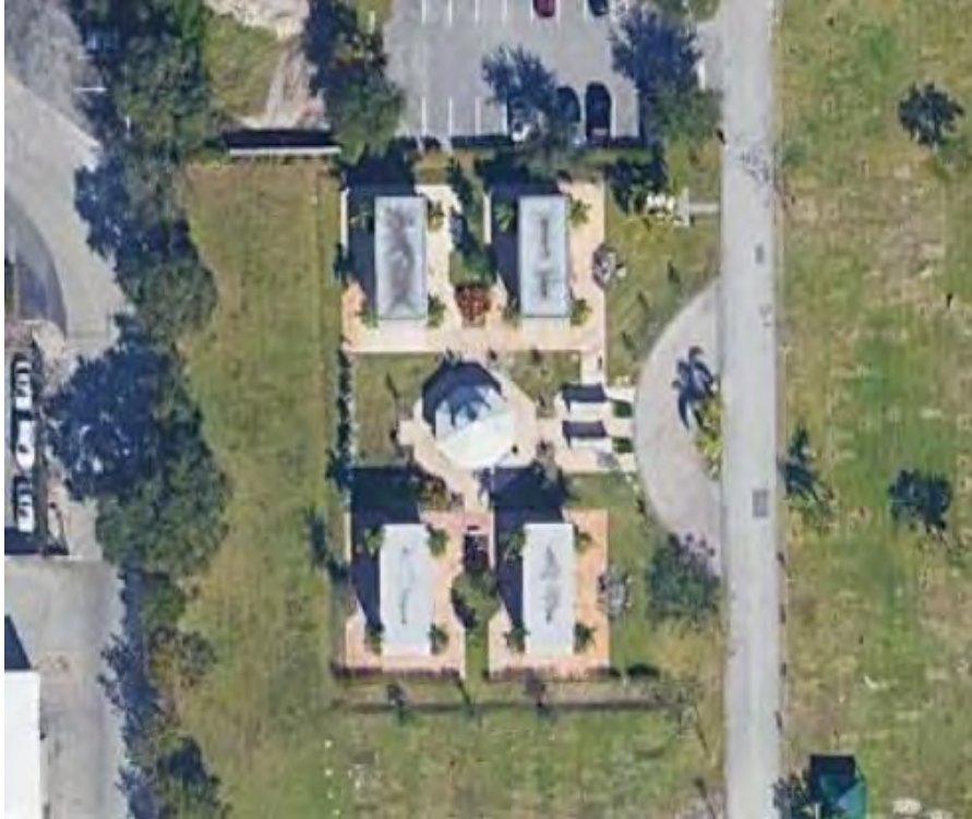
Aerial: West end of Cemetery – (4) Existing Mausoleum Buildings
