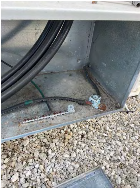
Picture 2 – Gutter Grounding Connections
