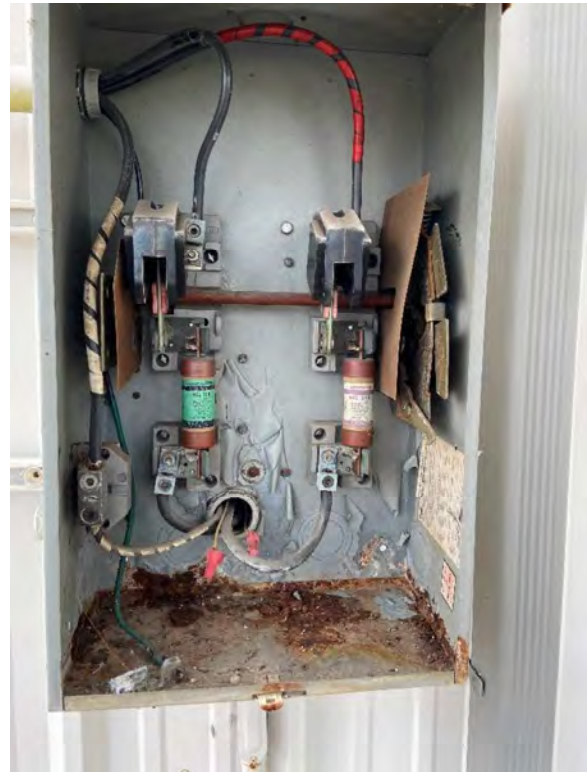
Picture 8 - No Main Bonding Jumper
