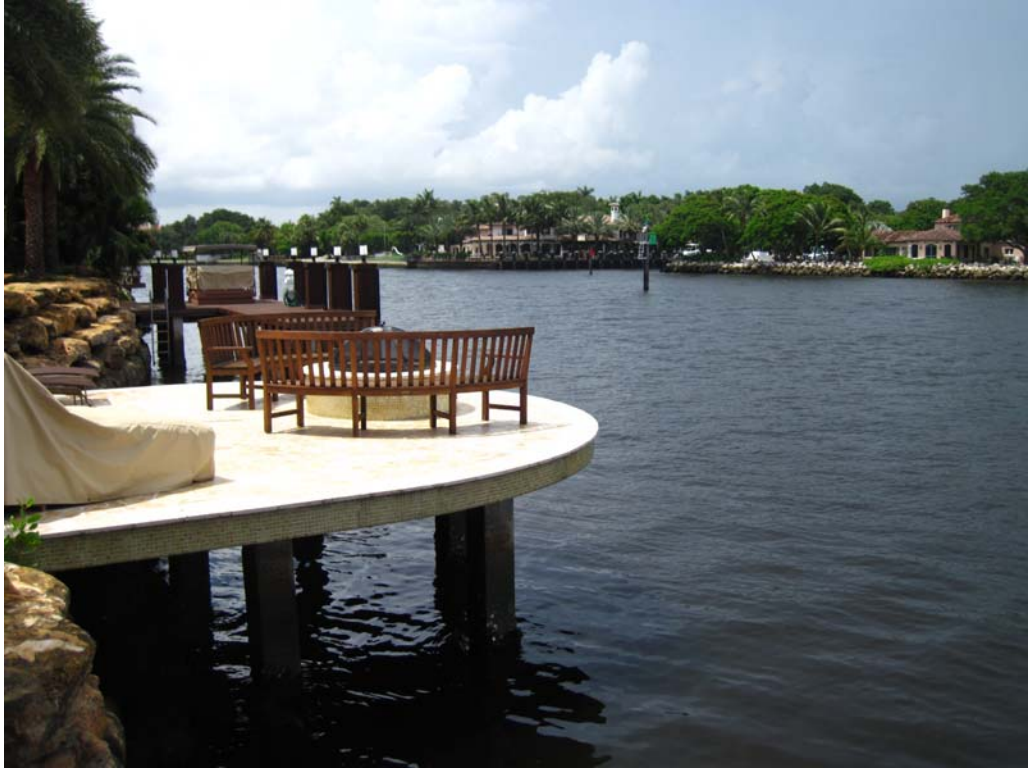
1. Western edge of property, facing west along the New River.
