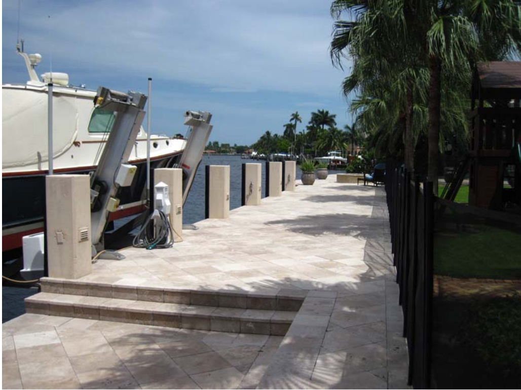
3. Western edge of property, facing east along the New River. Note: Existing dock and boatlift.
