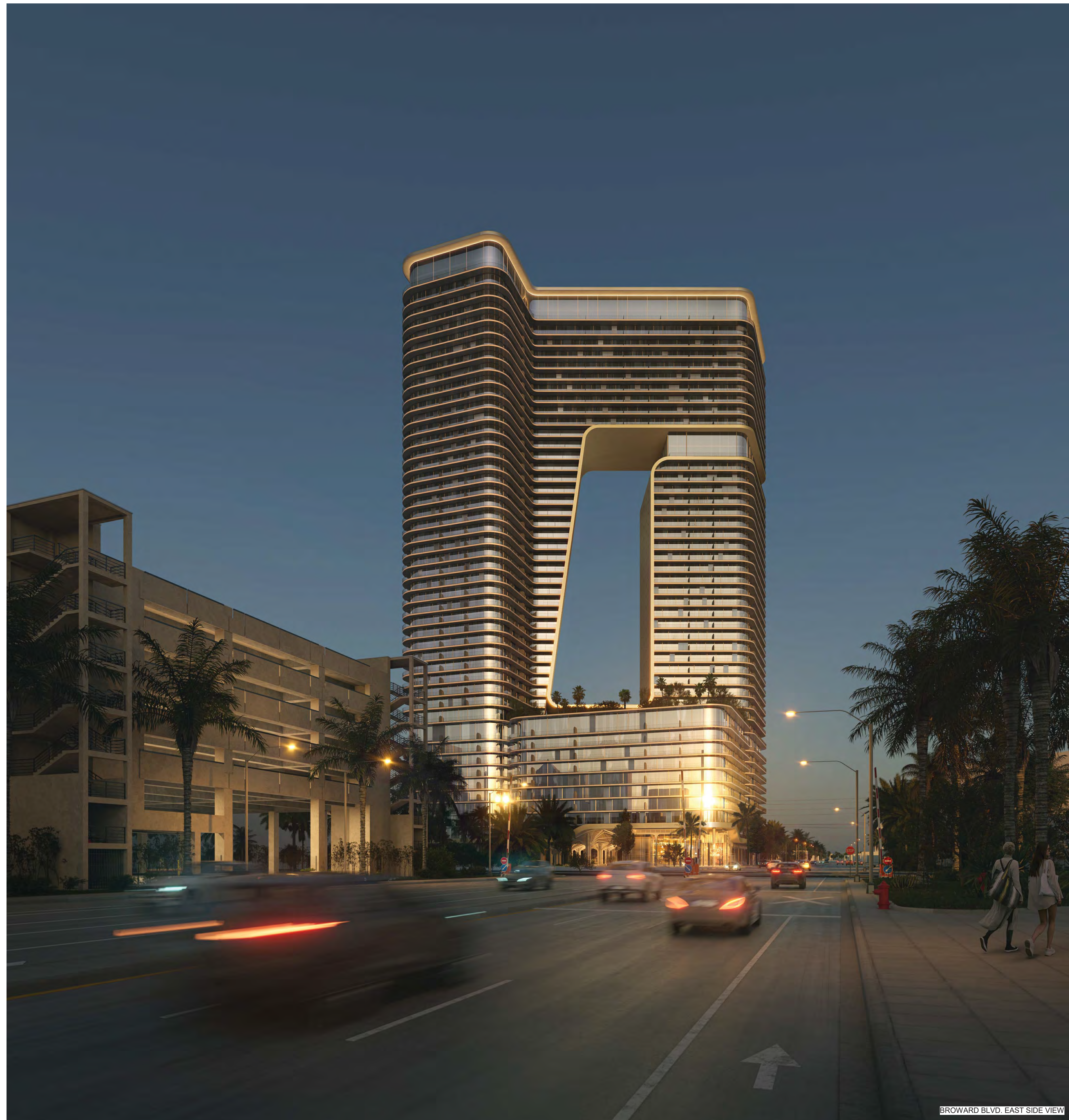
BROWARD BLVD. EAST SIDE VIEW
