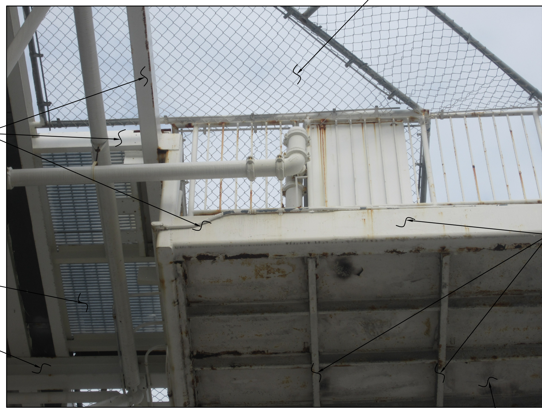
LANDING L-6 AND STAIR#7 PHOTO N.T.S. (5/S07)
