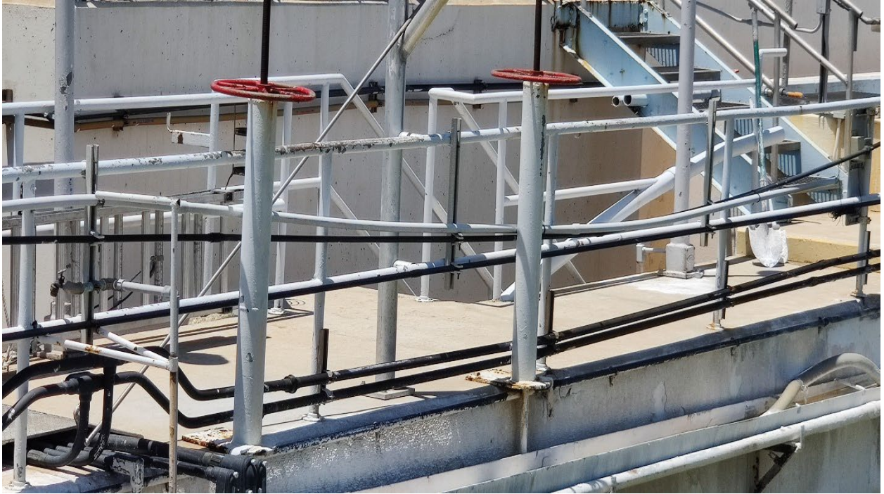
Gate #5: 98" W x 32" H, Steel frame mounted to wall, Hydro #1
