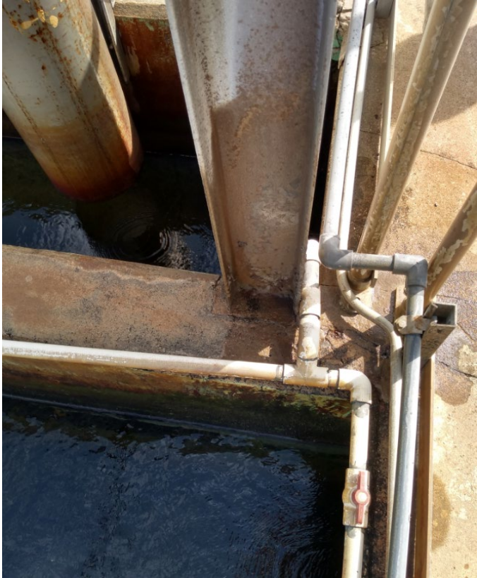
Gate #8: 33" W x 73" H Aluminum frame embedded in grout N.E. Corner Aerator Flume
