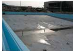
Aquatic Center, MDC North Campus, Buildings 15 and 40, Miami, FL
