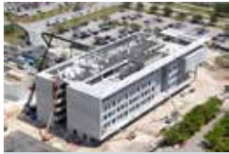
Classrooms and Student Services Building, MDC Kendall Campus, Miami, FL
