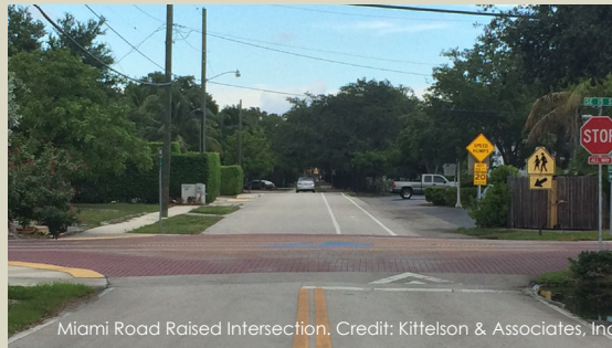
Miami Road Raised Intersection. Credit: Kittelson & Associates, Inc.
