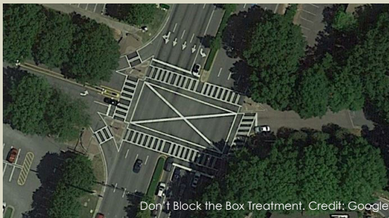
Don't Block the Box Treatment. Credit: Google
