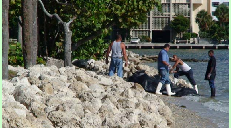
View of the Shoreline Stabilization Construction
